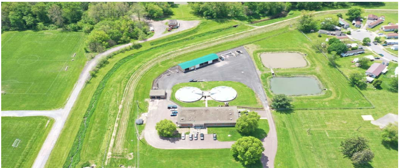
Aerial View of Danville Water Treatment Plant
